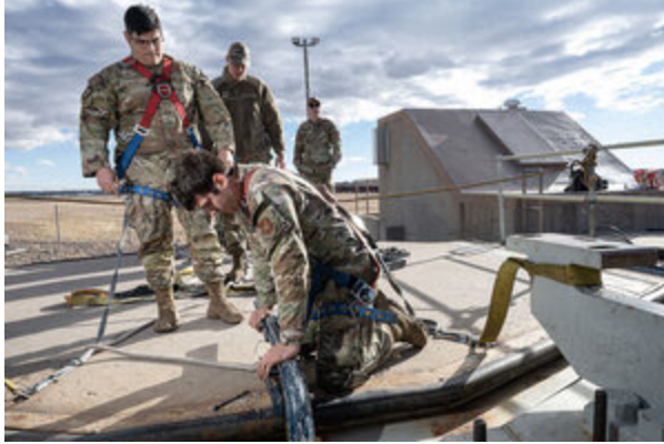
Air Force maintainers work on the launcher closure door for a Minuteman III at the training site. Alfredo Sosa/Staff
