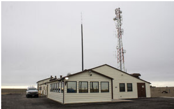
Missile Alert Facility Echo-01 in rural Kimball County, Nebraska.
